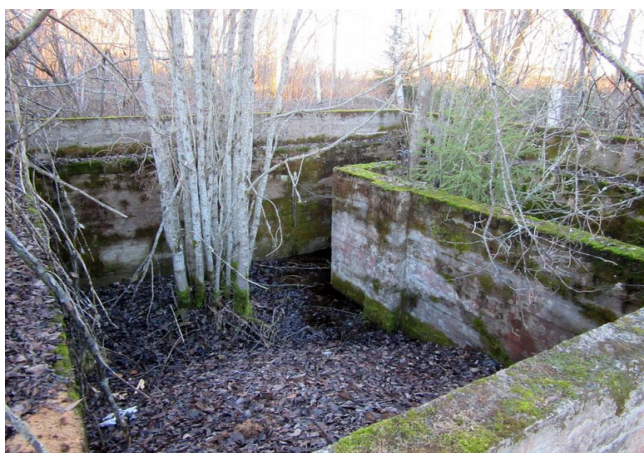
Kohde no. 2, betoniperustus.
